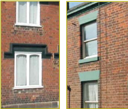
Figure 26: Illustration of some of the different window treatments within Halton Village: Timber casement with stone hoodmould; simple sash widow; leaded lights within stone subframe; small timber casements within timber framed building
