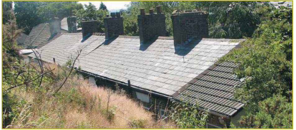
Figure 32: The effects of replacement roofs on the character of the village's roofscape
